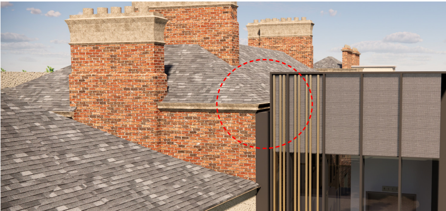
‘Shadow gap’ detail between lift core and existing eaves
